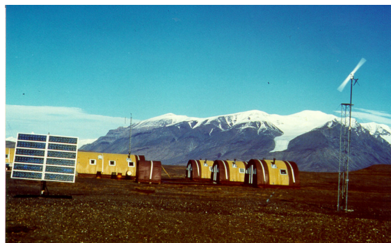
Figure 2: PV-wind-diesel hybrid system using tracker to power Parks facility in Tanquary Fiord, NWT
