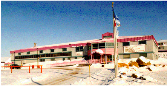
Figure 4: 3.2 kW p PV array mounted on the façade of the college and connected to the local electric grid in Iqaluit, NWT.
